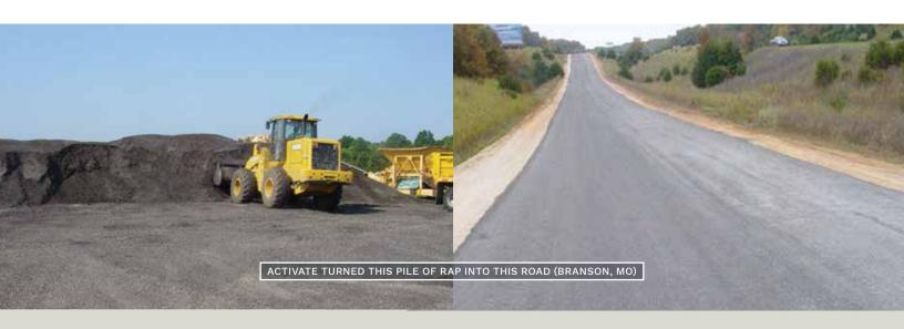
Activate restores Reclaimed Asphalt Pavement (RAP) millings to like-new asphalt ideal for potholes, edge ruts, shoulders, and other paved surfaces. Activate introduces new polymers to the mix while reducing oxidation in the RAP, creating an environmentally friendly surface built to last.
