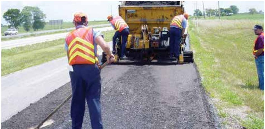
After Activate is mixed with RAP, it can be stored for two to six months. Larger piles, over 100 tons, of the mixture can be left uncovered while smaller piles can be covered with tarp. Stored mixtures stiffen over time, but a simple spray of Activate will soften the mix before use.
